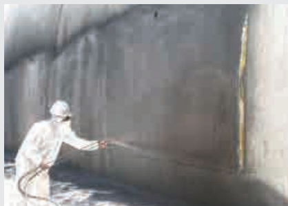
WATER PROOFING WALLS
